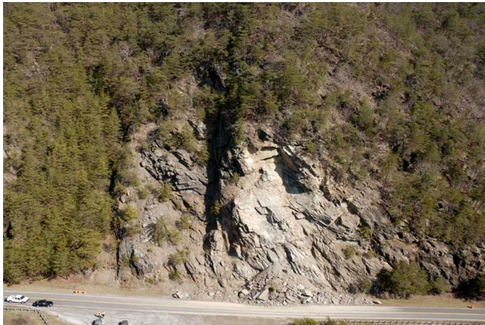
Aerials of rockslide on US-129.
